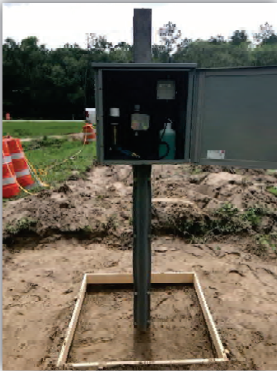
Custom Remote Settlement Cell Monitoring Station at an Active Sinkhole Location
