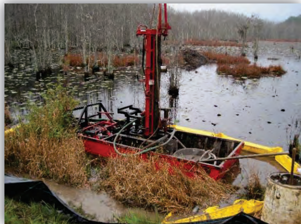
EGS “Swamp Skid” in Action
